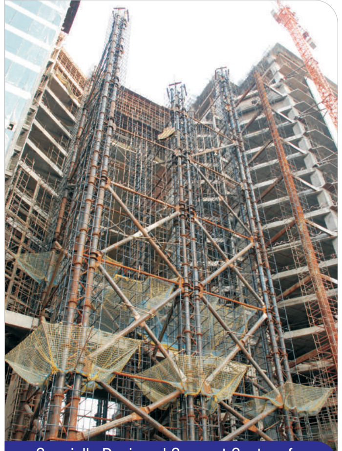
Specially Designed Support System for casting the Suspended Slab at 34th Floor
