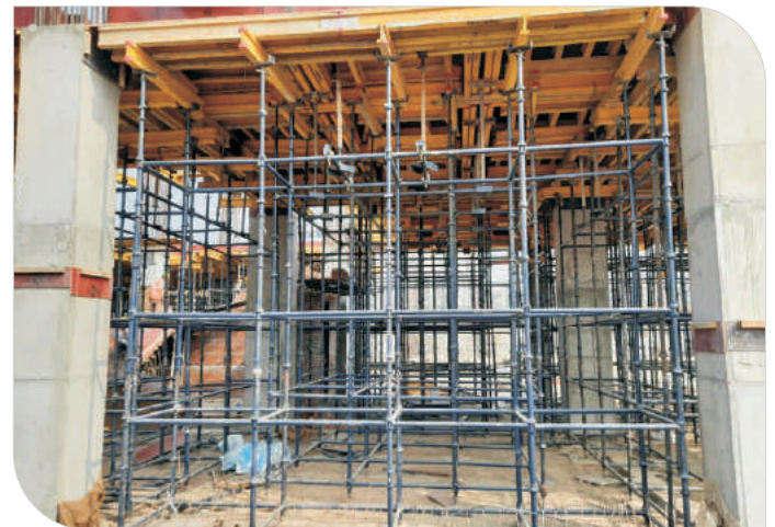
Specially Designed Support System for casting the Suspended Slab at 34th Floor
